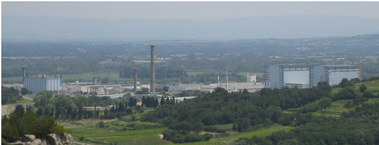
Marcoule Nuclear Centre, France, where plutonium was produced for military purposes until 2009.
