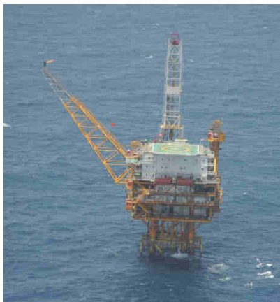
2nd structure: observed in July 2013
