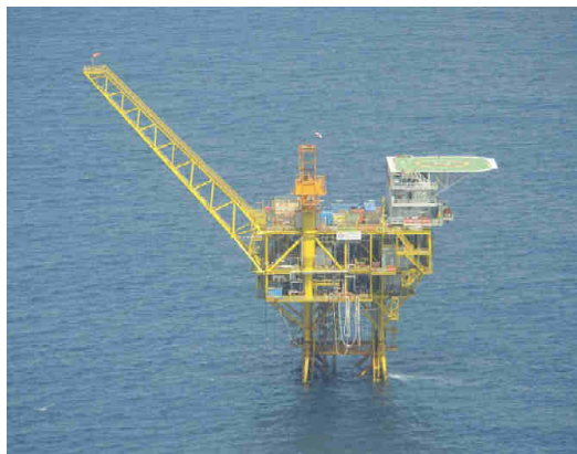
4th structure: observed in April 2014
